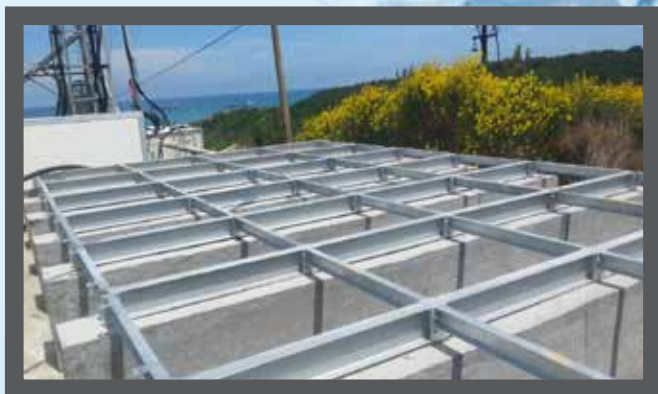
05 Steel Skid Installation on Concrete Base
